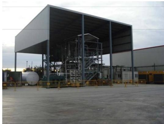
Fig 4 Alphakat 2,000 liter/hour synthetic diesel plant
